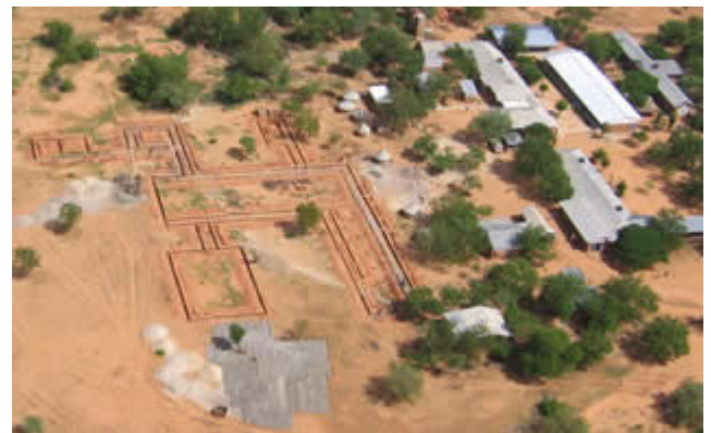
Foundation of 42-bed Fistula Clinic being built in Niger
